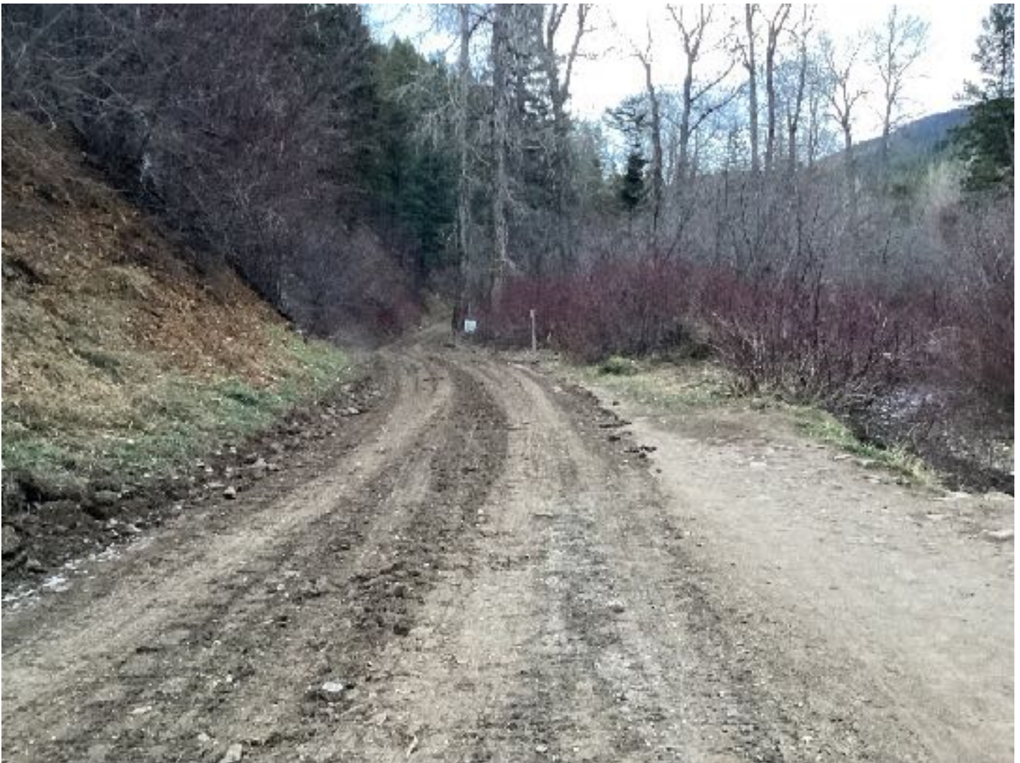
Figure 1 The Sourdough Trail is open and blading and remediation has been complete for the winter.
